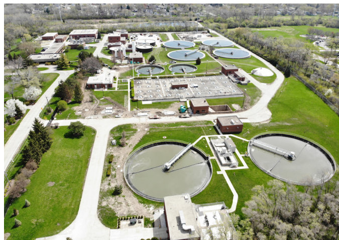
Aerial view of GWA's Advanced Wastewater Treatment Facility. Photo credit: Glenbard Wastewater Authority
